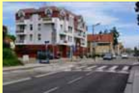
Route de Lyon © egis rail-c.dereymez
